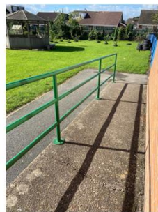
The external ramp connecting the hall, N/R/Y1 to the outside area.
